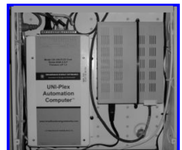
The C2k1 UNI-PLEX Automation Computer, manages the complete system
